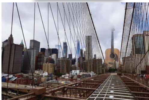
02 - Brooklyn Bridge Revisited.jpg
